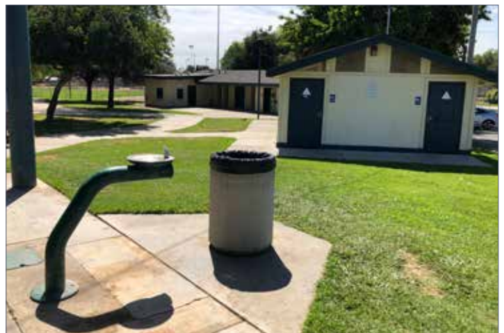
Restroom facility at park
