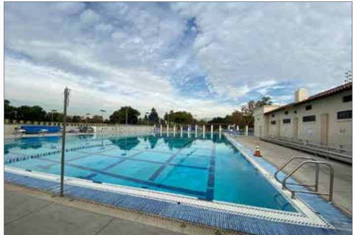
George Hansel Aquatic Center at Montebello City Park
